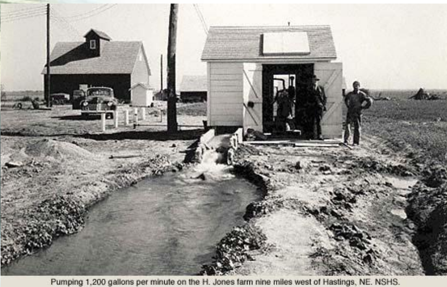
Pumping 1,200 gallons per minute on the H. Jones farm nine miles west of Hastings, NE. NSHS.
