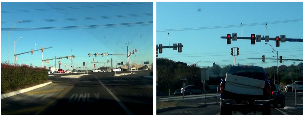
(a) Triple right-turn lanes on the eastbound approach (RTOR allowed)
