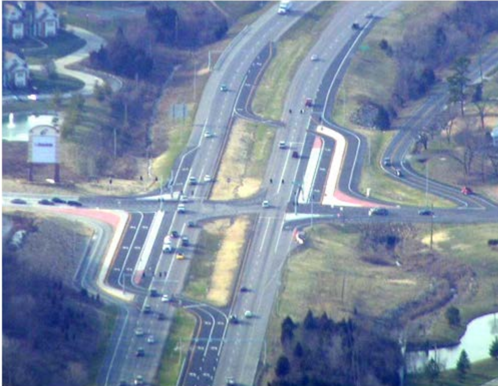
Figure 8-2. A CFI Intersection in Fenton, MO.
