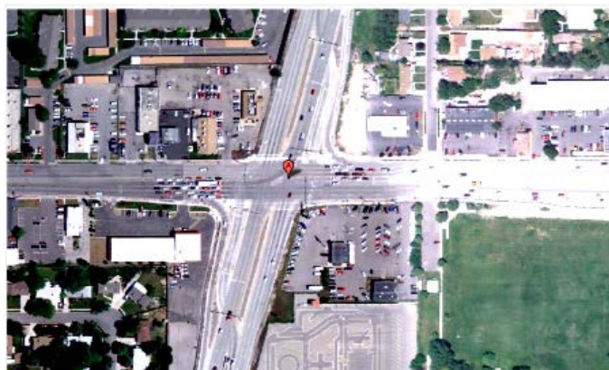
(b) Aerial photo of a CFI intersection, 3500 S & Bangerter Highway, Salt Lake City, UT
