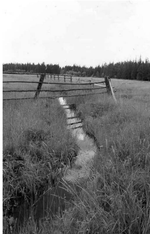
Figure 3. A field canal dug in the Soviet period to drain hay fields.
